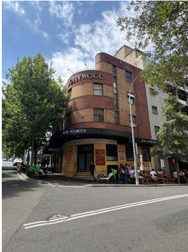
Figure 1: 2 Foster Street, Surry Hills, viewed from the north-west
